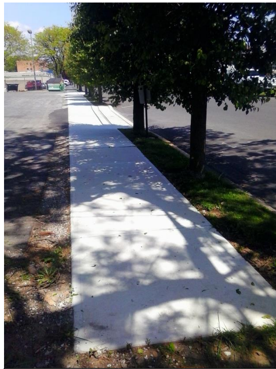
Figure 13: New sidewalk in front of the Borough Authority on Front Street.
