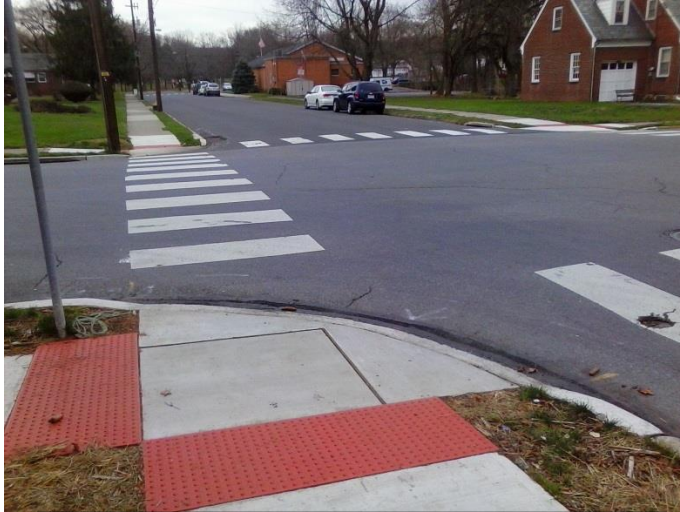
Figure 10: New ADA-Crosswalks at the Water and Northampton Street Intersection
